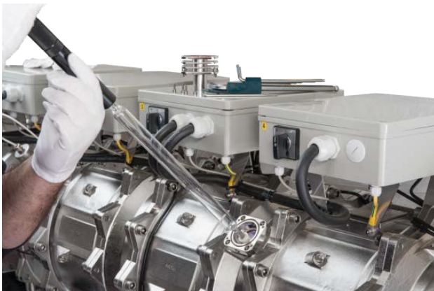
Two Lamp Unit Bulb Replacement
